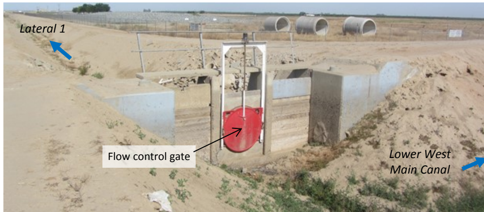
Figure 36. Existing Lateral 1 flow control headgate on the Lower West Main Canal
