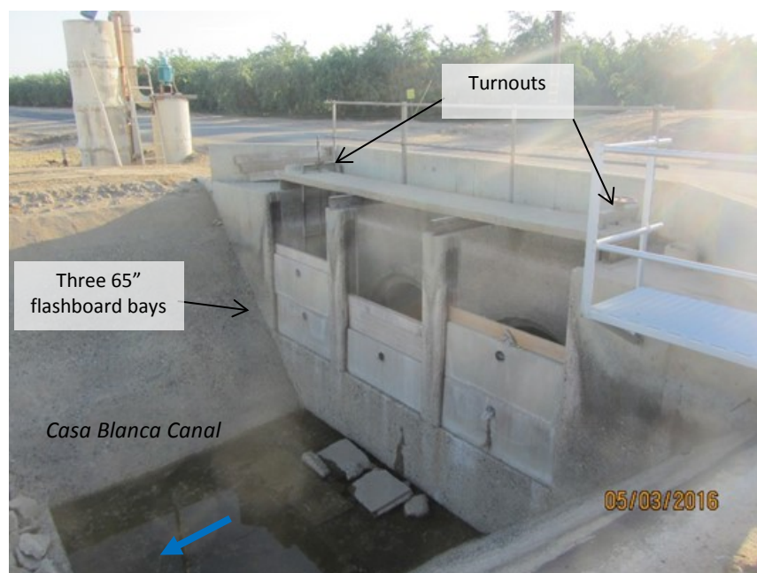
Figure 20. Check structure in the Casa Blanca Canal, just downstream of Avenue 116 Canal entrance
