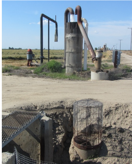
Figure 5. Typical conjunctive use system in PIXID. A well pump (on the left) is discharging into a standpipe. A low lift pump (right side) will lift canal water into the same standpipe.
