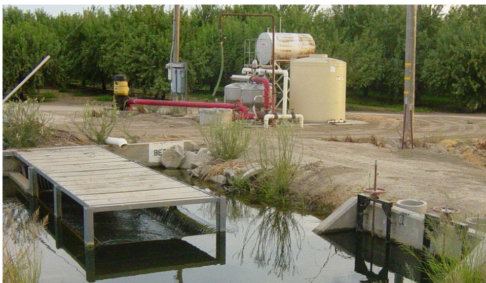
Figure 13. Retrofitted long-crested weir at Chowchilla ID
