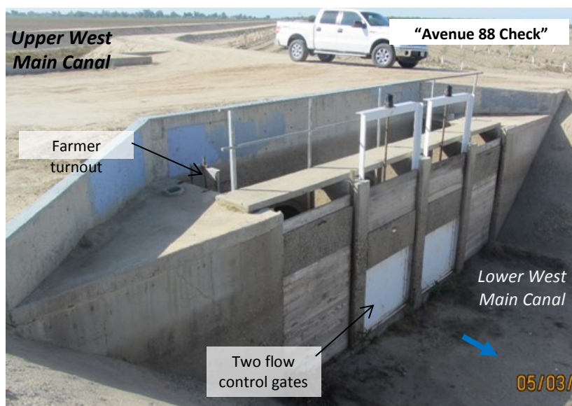
Figure 31. View “C” from Figure 28. Avenue 88 Check; Flow control gates at the entrance to the Lower West Main Canal
