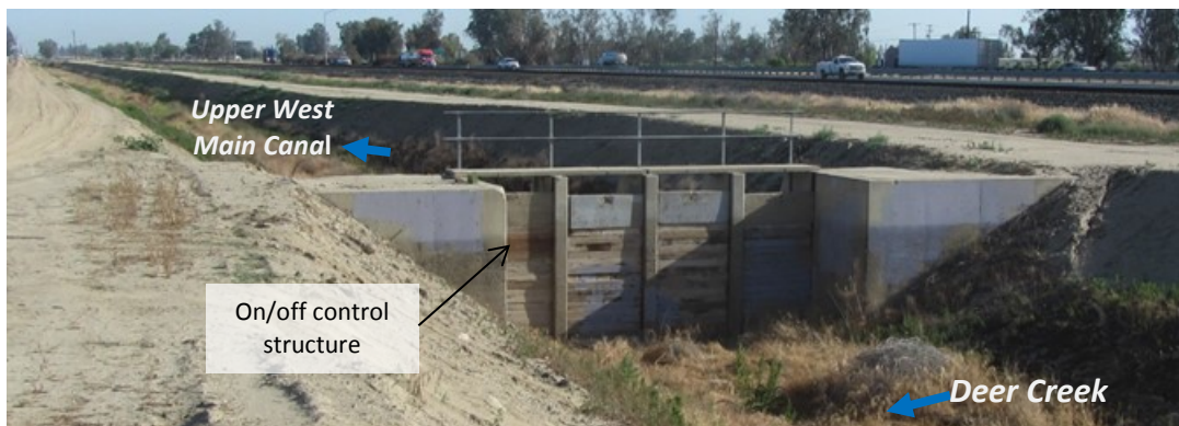
Figure 30. View “B” from Figure 28. Existing structure at the head of the Upper West Main Canal used for on/off control. During the irrigation season, the structure is wide open.
