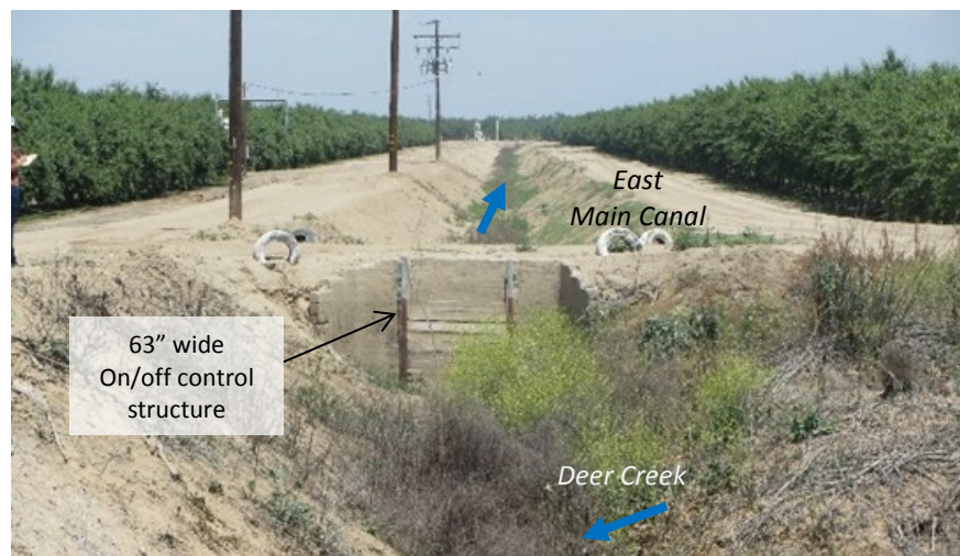
Figure 25. Existing structure at the head of the East Main Canal used for on/off control. During the irrigation season, the boards are removed.
