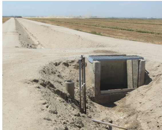
Figure 6. Typical check structure and turnout on the North Canal. Typical flow rate is 15-20 CFS.
