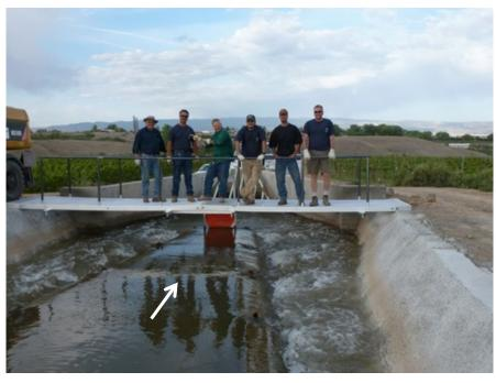
Figure 30. Example long-crested weir pointed downstream. District (un-named to protect the guilty) employees are performing a structural test on the bridge used to access the flushing gate.
