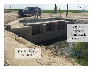
Figure A-17. Location B from Figure A-15. Existing flashboard structure that maintains water level in the Westside Intertie before spilling into Canal 2 through two pipelines. Photo looks to SW.
