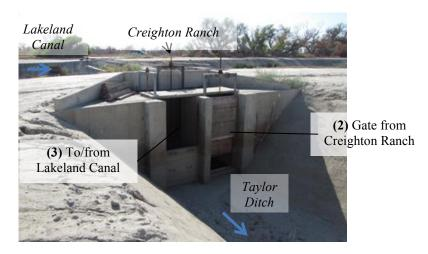
Figure B-4. Location A from Figure B-3. Gates at head of Taylor Ditch.
