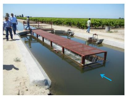
Figure B-26. Example design for long-crested weir at Site 4 in Taylor Ditch (upstream facing)
