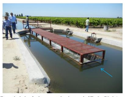
Figure B-46. Example design for long-crested weir at end of Taylor Ditch (upstream facing)
