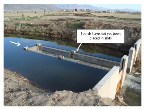
Figure 29. Example simple long-crested weir pointing upstream. Walker River ID, Nevada.
