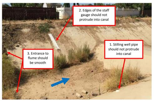
Figure 26. Recommended modifications to Woods Central Canal Replogle Flume
