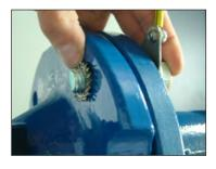
**STEP 7**Add serrated washer to the other side of the bolt (on meter's flange side).
