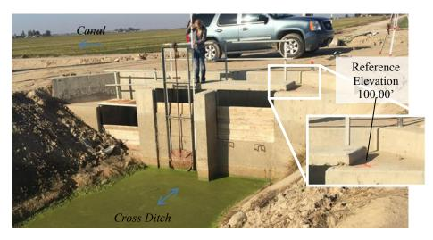
Figure A-26. New operation at the bifurcation of Canal 2 and the Cross Ditch
