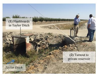
Figure B-23. Location B from Figure B-21. View to SE of check structure and turnout at Site 4 on Taylor Ditch.
