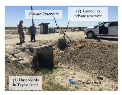
Figure B-22. Location A from Figure B-21. View to SW of check structure and turnout at Site 4 on Taylor Ditch. Private reservoir in background.
