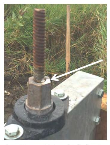
Figure 6. Proper cut in shaft to mark the "zero" opening
