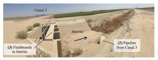
Figure A-11. Location C from Figure A-8. View toward SE of the Intertie after flowing under Canal 3 (Canal 3 is shown on left).
