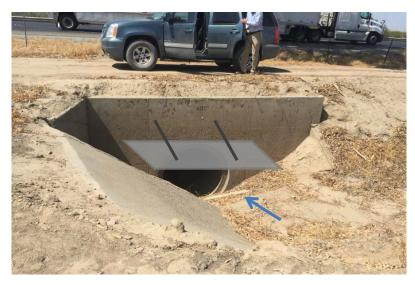
Figure 22. Example layout of vortex suppression plate on upstream side of culvert
