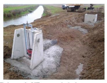
Figure 16. Final concrete for GCID metergate, showing downstream pre-cast outlet box
