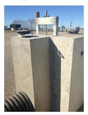
Figure 13. GCID metergate at Briggs
