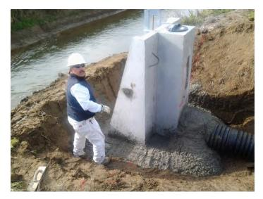
Figure 15. Installation of GCID metergate
