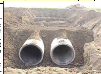
Double Barrel 60" Pipe Under Lateral #3
