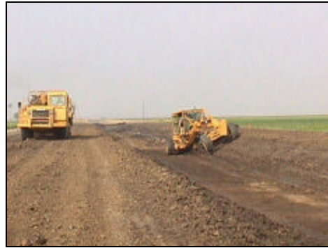
Excavation and Shaping of Inter-tie Canal from Lateral #4 to Lateral #3
