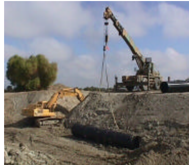
Pipe Replacement at Creighton Ranch
