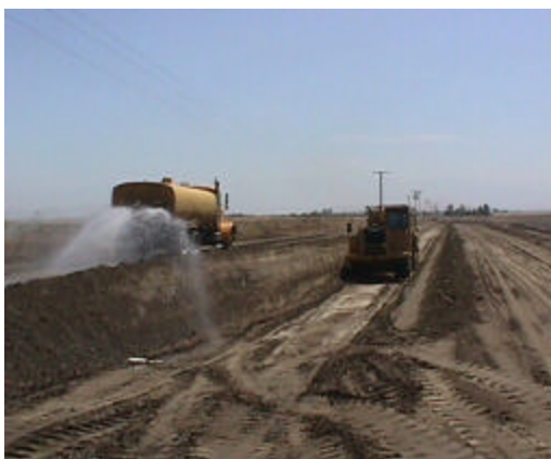
Moving dirt and applying water
