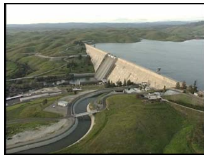
Millerton Lake behind Friant Dam
