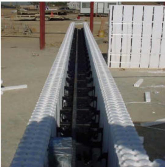
Below Left: Half section of Insulated Concrete Form with horizontal steel support. Vertical steel support added later
