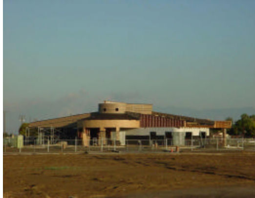
Above Right: View of construction in early November.
