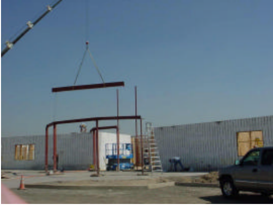
Above Left: Crane sets steel for entryway. The vertical steel is encased in five-foot diameter casings eight feet deep.
