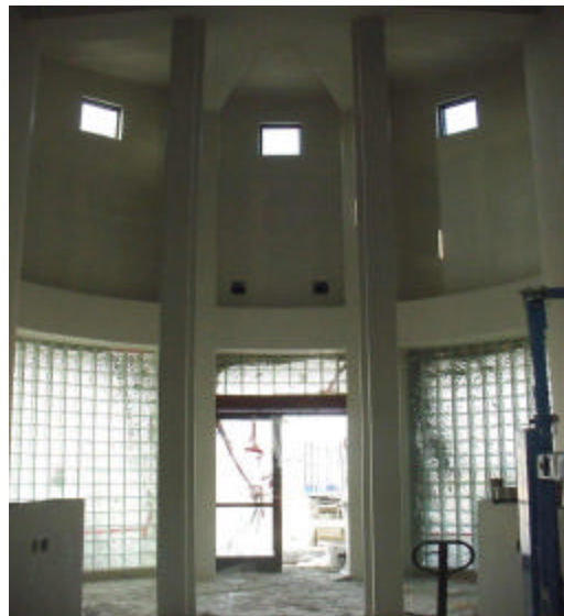
Below Right: View of unfinished interior entryway. Ceiling heights total more than 25 feet to accommodate roof slope
